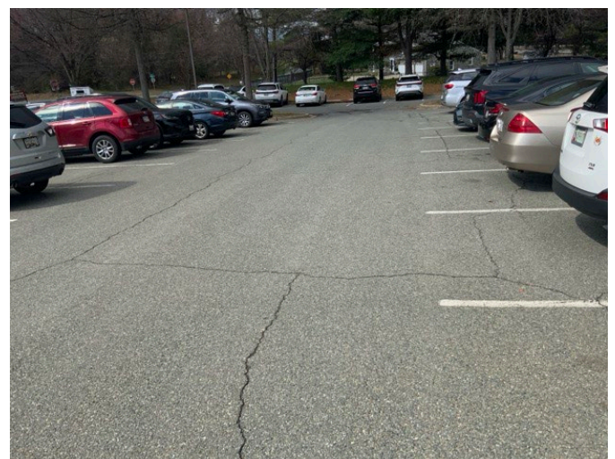
30 - ASPHALT PARKING LOT
