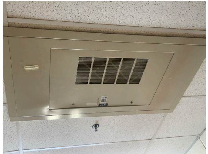
14 - CEILING MOUNTED UNIT HEATER
