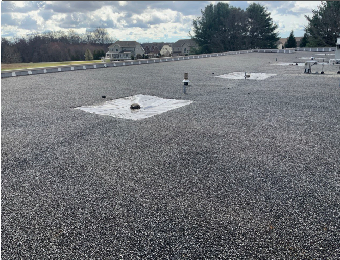
7 - BUILT-UP ROOFING
