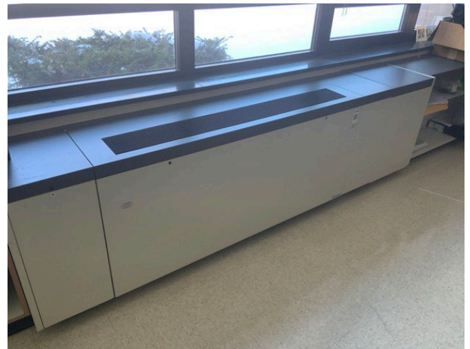
16 - UNIT VENTILLATOR
