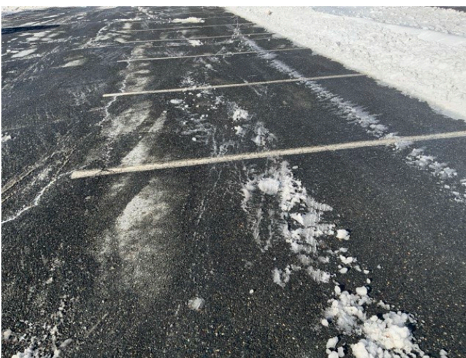
29 - ASPHALT PARKING LOT PAVING
