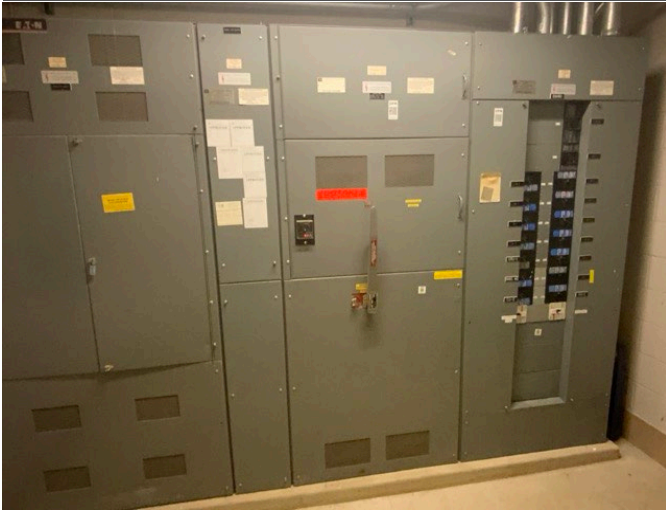
25 - ELECTRICAL SWITCHBOARD
