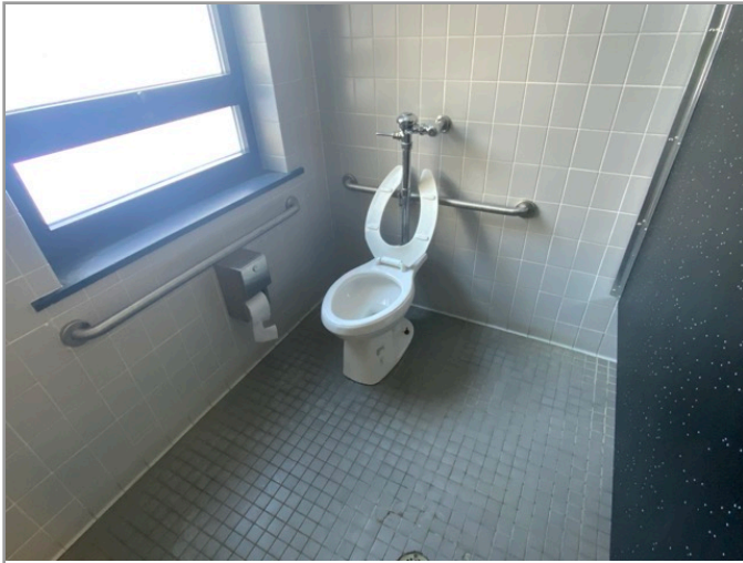
TOILET STALL OVERVIEW
