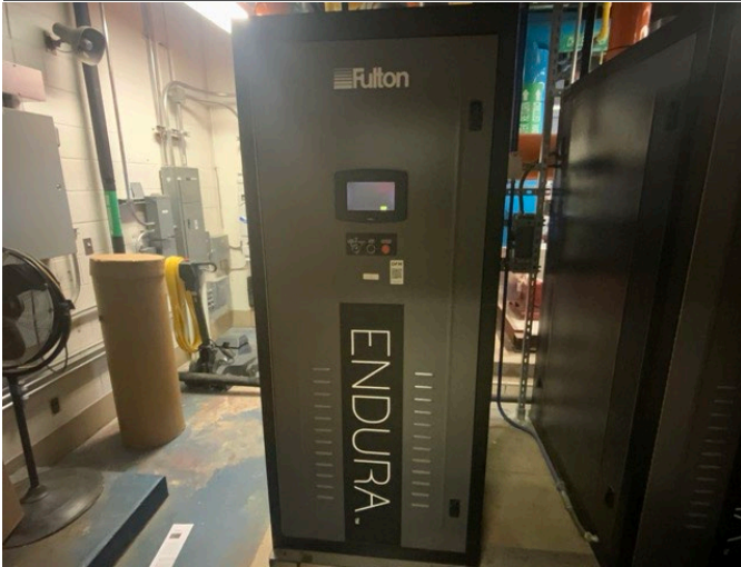
13 - CONDENSING BOILER
